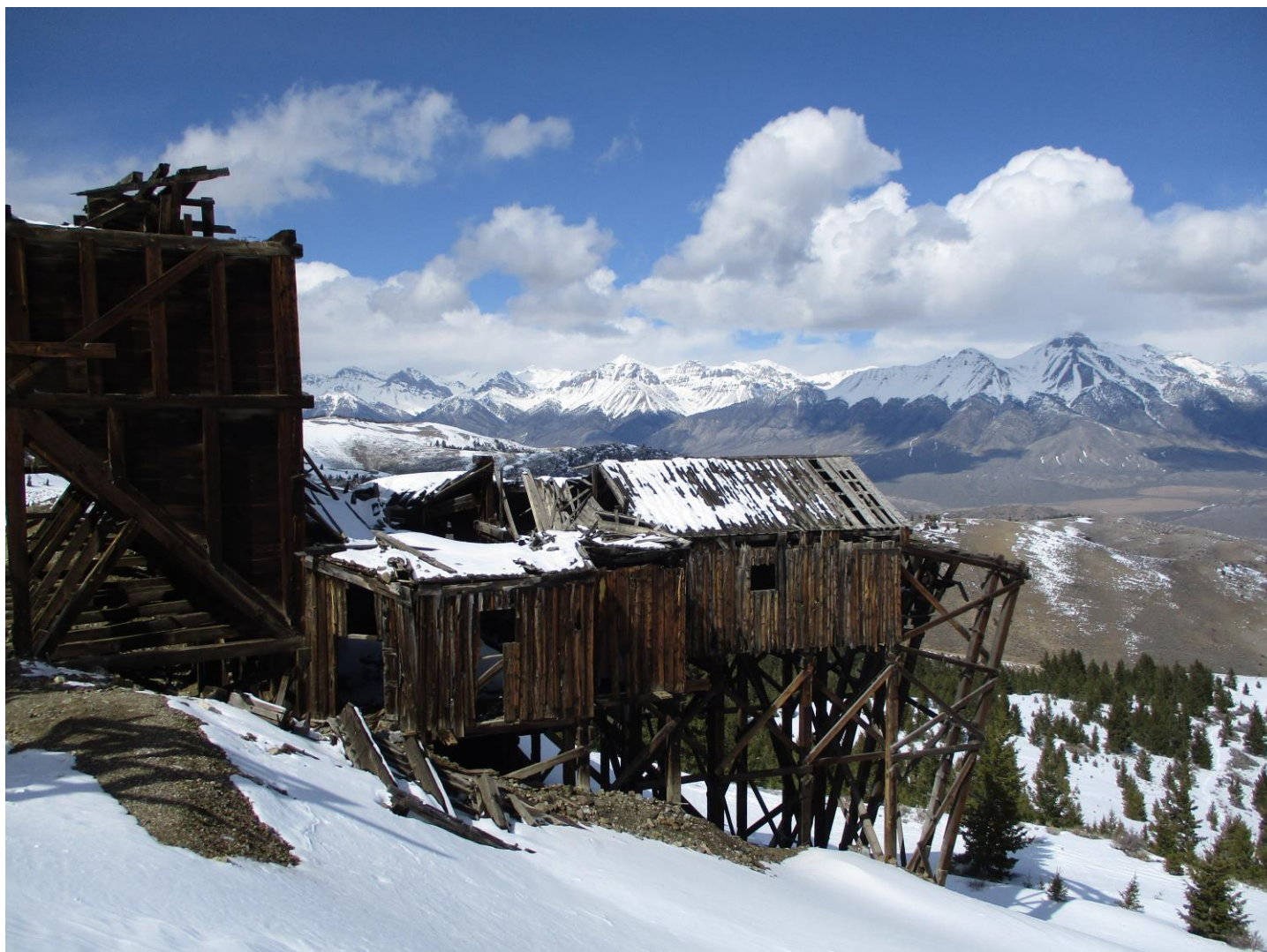
Mine workings from an earlier phase of mining at Empire
